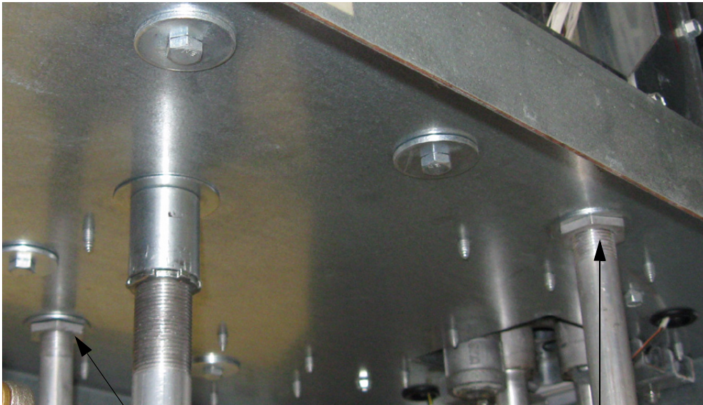
Valve Conduit Nut and Washer, typical
